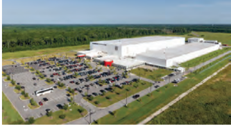
MHPS' Savannah Machinery Works is the comprehensive manufacturing, service and repair center for gas turbines, steam turbines and generator rotors.
